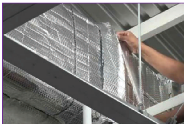
Ductwork Class 1 insulation with aluminium foil.
